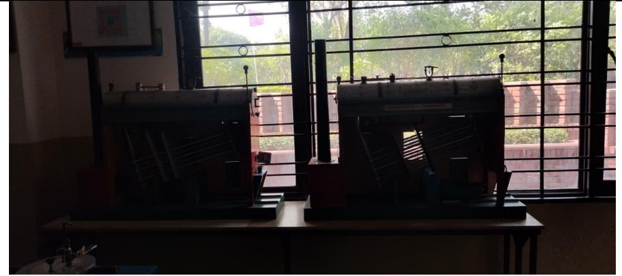
P-30 | Cooling Tower Date: 25-04-2026 | Geotag: NOT AVAILABLE (no GPS EXIF)
